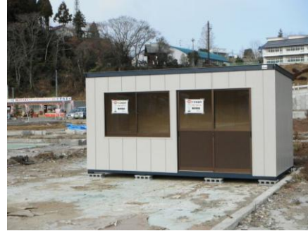
A temporary bus stop in Minamisanriku, protecting the users from strong coastal winds and snow as the temperature stays below zero Celsius in this region. ©JRCS
