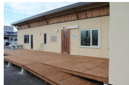
Community centre for Kawauchi built in Koriyama where the villagers are evacuated. The centre is designed to be mobile and will be relocated to Kawauchi once the village is ready to move back. ©JRCS
