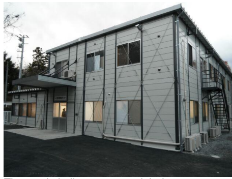
The newly built temporary night-time emergency medical centre in Ishinomaki; a steel-framed two story temporary building. ©JRCS
