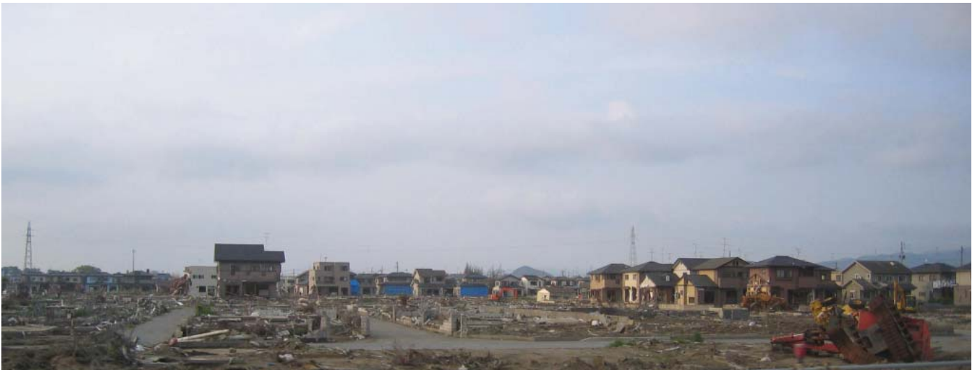
Scene of destruction in Ishinomaki City – houses missing from foundations; those standing are no longer habitable.
