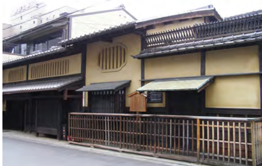
The Noguchi Machiya – a Kyoto machiya used as a private residence. The mushiko mado can be seen on the second floor.
